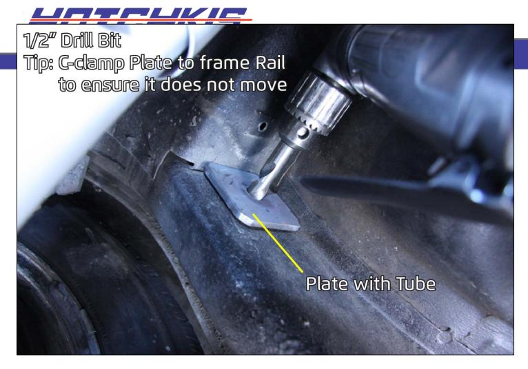
Note: In some cases, you may need to relocate the fuel line if they are in the way when installing your frame mounts. You should be able to easily bend the lines out of the way and relocate the adel clamps that hold them in place.
